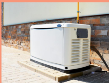
BACKUP PLAN: Standby electric generators—either portable or permanently installed, like the one pictured—can power essentials (or even entire buildings) during outages
